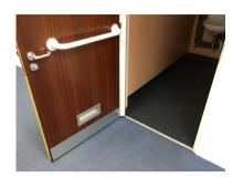
2.6.2.2 The cubicle door achieves a clear width of around 870mm which should be adequate for all users.
