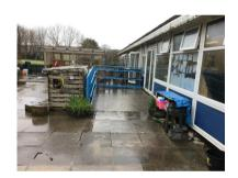
3.1.8.2 The ramp is generally well detailed achieving a suitable gradient with ergonomic handrails to either side, a reasonable width and what appears to be adequate lighting.
