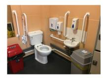
2.6.2.4 The cubicle is set out in a corner layout designed for independent use. It is generally well detailed and should prove accessible to most users.
