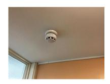
2.14.2 We are pleased to note that accessible toilets appear to be fitted with beacons linked to the fire alarm to give additional warning to a hearing impaired user.
