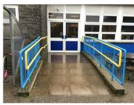
2.1.4.1 The ramp to Year 3 is generally well detailed achieving a suitable gradient with ergonomic handrails to either side, a reasonable width and what appears to be adequate lighting.
