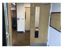
3.4.1.2 The internal doors are generally well detailed with ergonomic ironmongery including tubular lever or pull handles.
