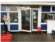
with an approximate level change of 250mm posing a barrier to a wheelchair user or those unable to manage steps.
